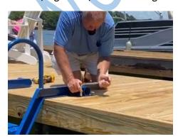
Note: When putting on the foot with the hole and yellow sticker, be sure you place the loop of the locking pin under the washer/lag screw before tightening. This IS IMPORTANT – it will keep you from losing your locking pin or it going into the water. It should be in the outer position. (Pic D)
